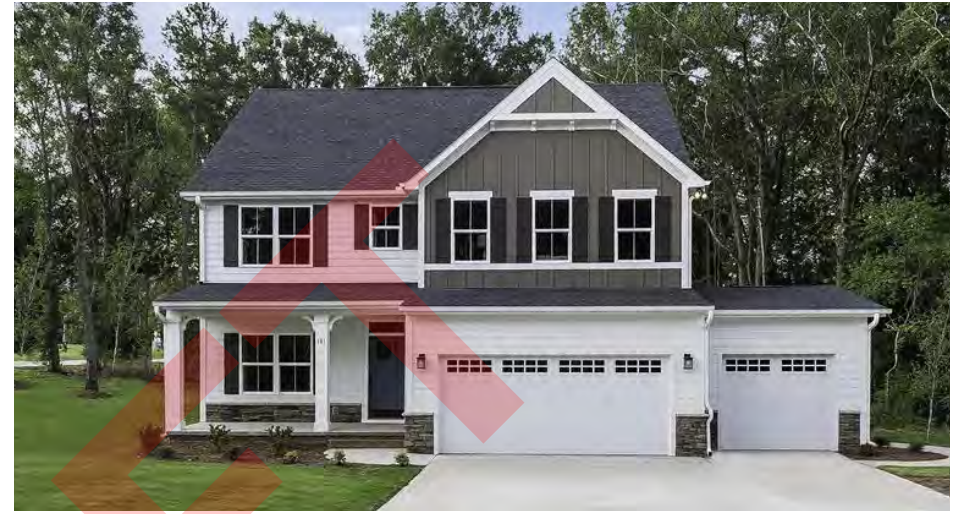
W New two-story single-family home at the Briar Creek Estates Subdivision in Whiteland. Source: Ryan Homes.
