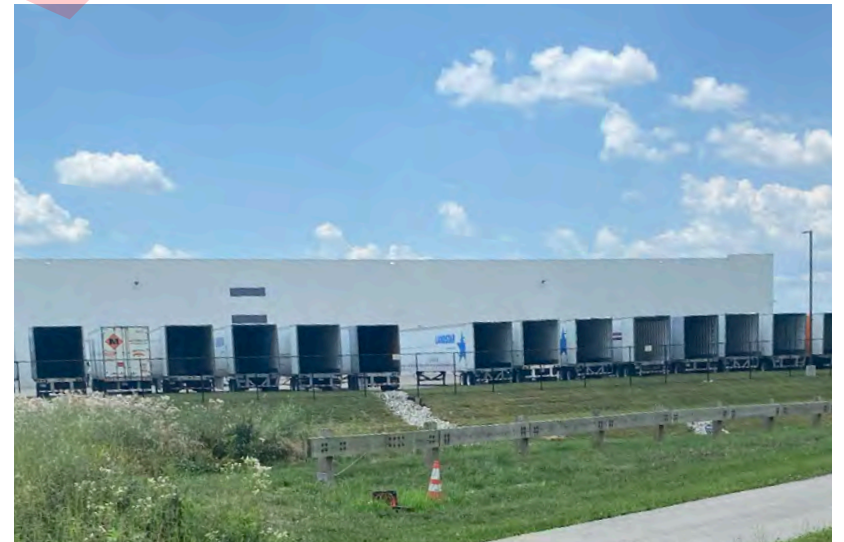
W View looking west towards industrial facilities. Source: Context Design.
