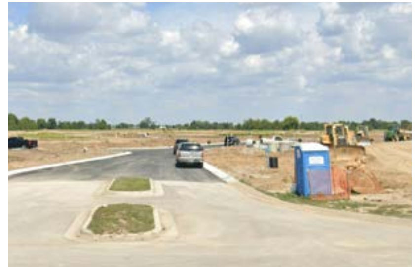
W View from Main St. looking towards the parcels. Source: Context Design.
